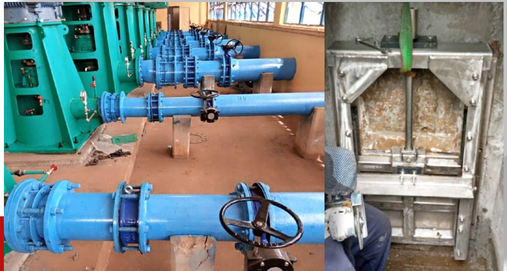
Ductile iron fittings, pipes, valves and penstocks for Ero Dam Water treatment plant rehabilitation 2020
